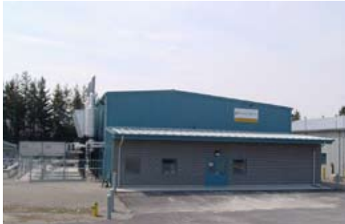
The 2.5 MW Guelph Hydro power plant was built in just eight months to meet the requirements of Ontario's renewable energy program.
